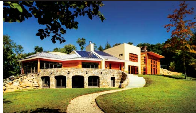
The home steps up a 20-foot slope at the rear of the site. Stone and wood were reclaimed from the property for such diverse uses as the exterior walls and the 14-foot-long table in the dining room.
